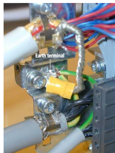
Figure 6.g - Cable installation in Carel NXL, MF2 (500V, 3-phase)
